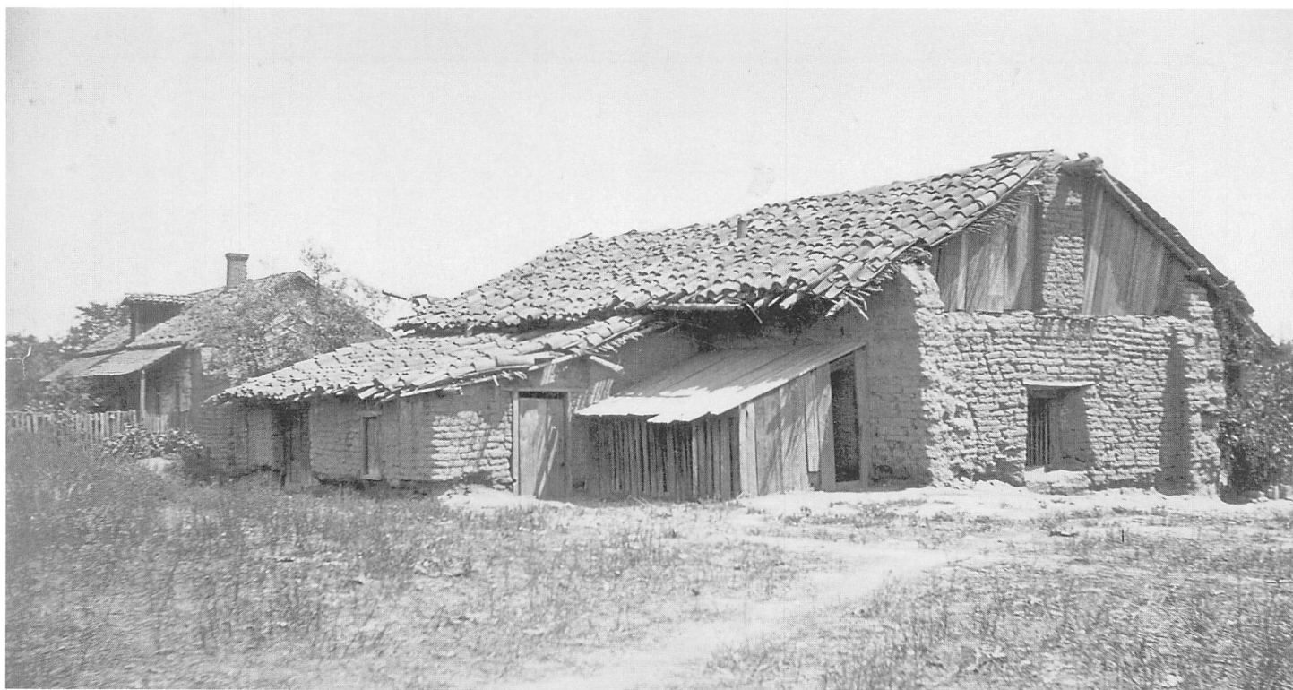
Adobe dwelling similar to those found throughout California in the early part of the 19th century. This one was near Mission Santa Clara, photograph by Fiske, circa 1875. Courtesy of the California Room, San Jose Public Library.
